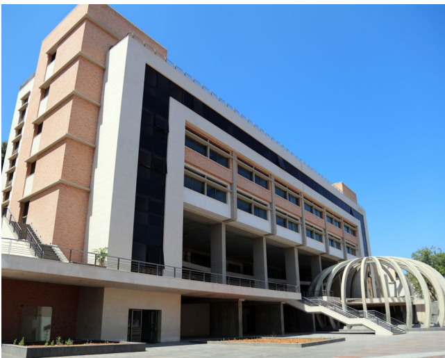
Under Construction: Faculty of Engineering and Technology Building, Hadat–Baabda Campus
